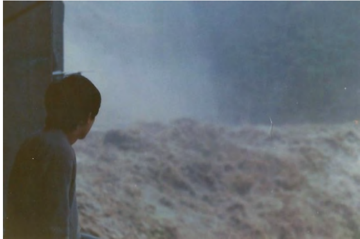
堰堤の肩を越える濁流
